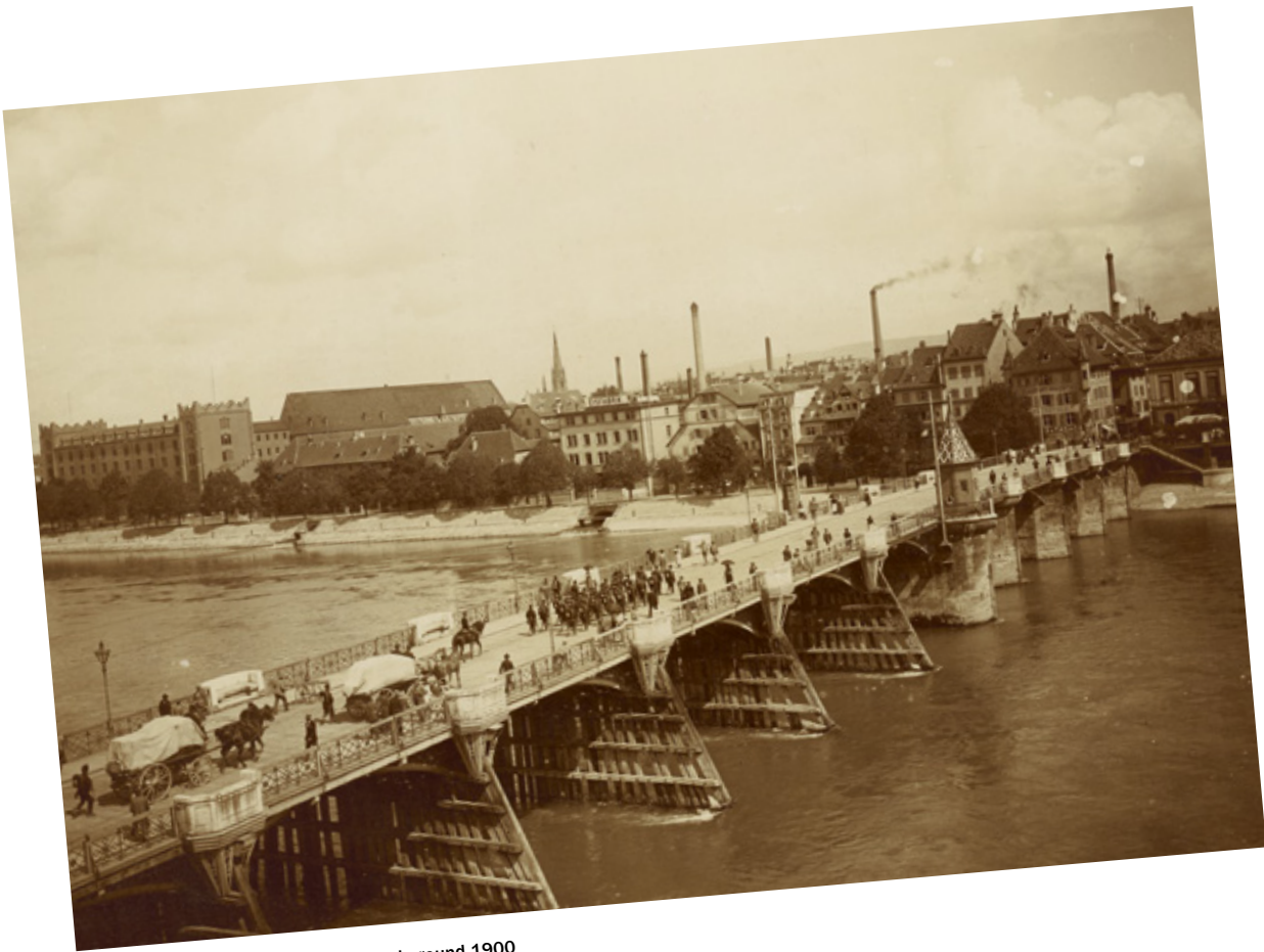
The old, partly wooden 'Mittlere Brücke' around 1900 Picture: Staatsarchiv Basel-Stadt. BILD 1, 64
